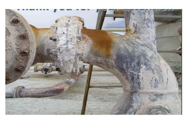
Fig. 2B: Example of mineral deposition at Soultz: Dissolution of material in the reservoir and re-precipitation at shallower levels may reduce flow in the reservoir close to the well and in the well and tubing and can cause serious damage to the equipment.
