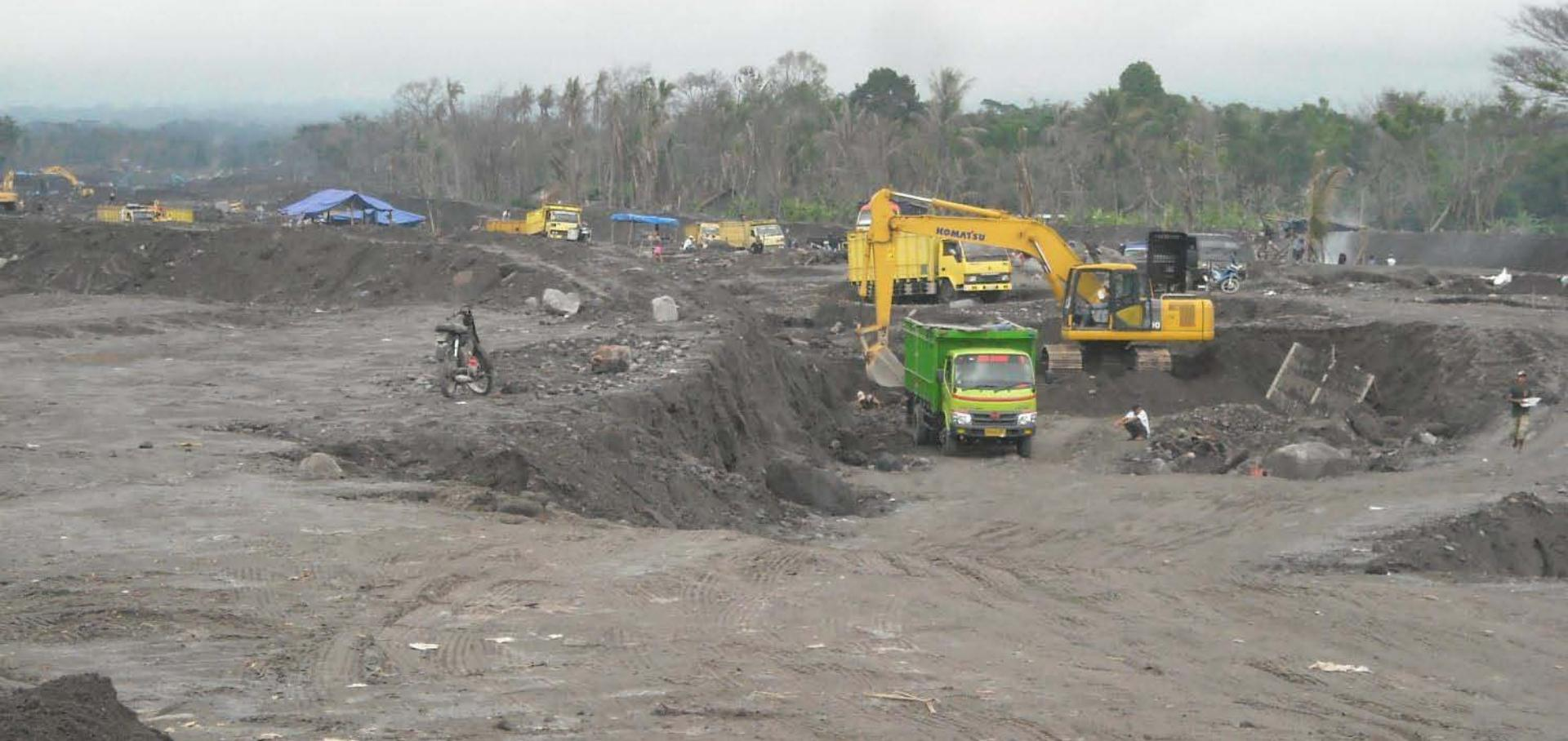
Some channels totally filled by pyroclastic flows => need artificial path needed for lahars
