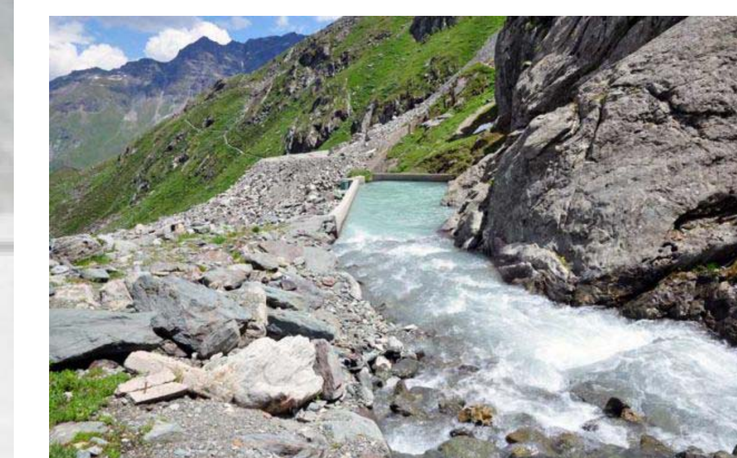
Fig. 5: Water intake (left: upstream, right: downstream) of Grande Dixence, illustrating the problem of zero flow conditions (Source: www.pronatura.ch )
