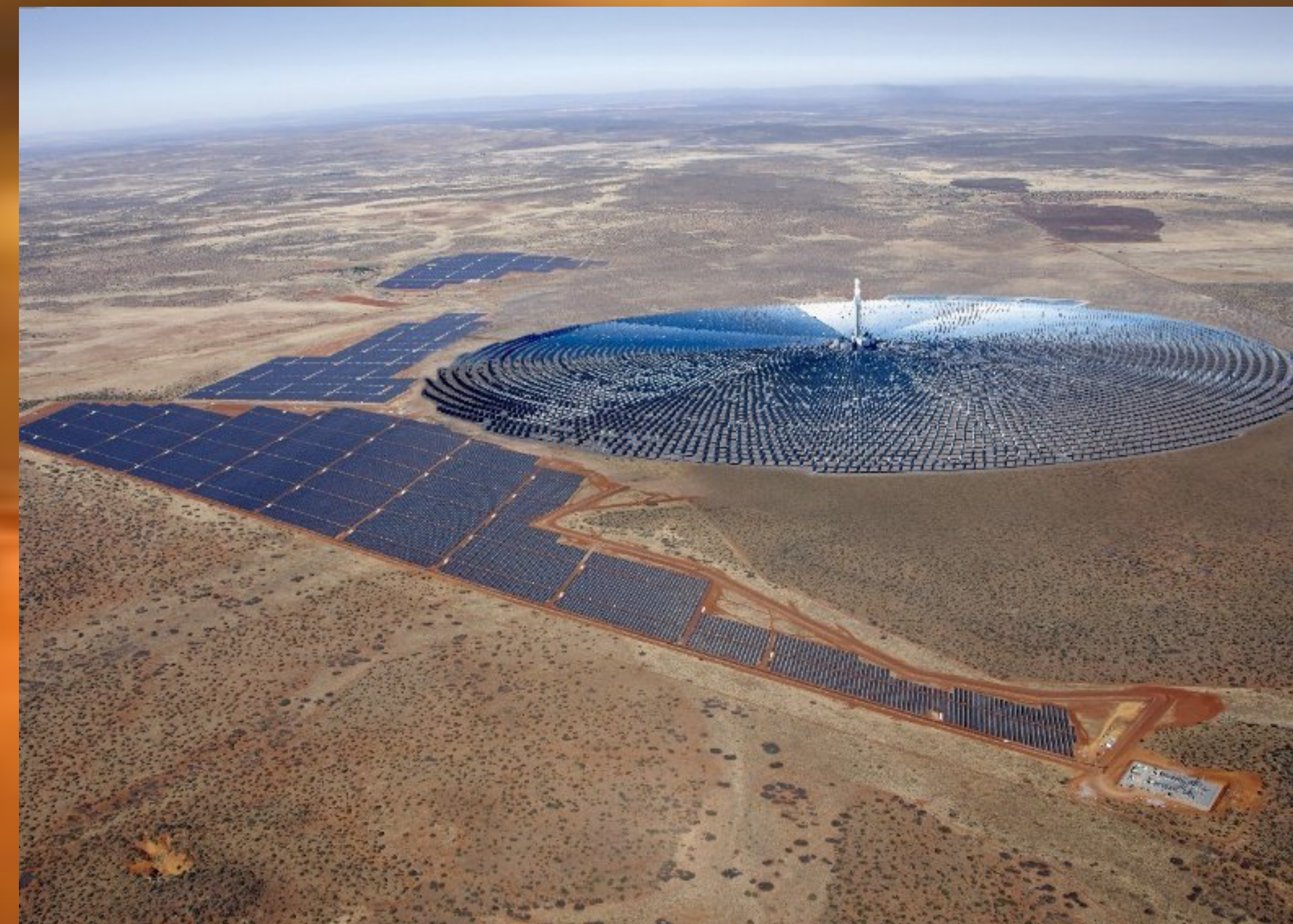
Figure 1 SolarReserve's Redstone 100 MW tower CSP with 12 hours of storage in South Africa sited next to their three PV projects, Lesatsi, Lesedi and Jasper. Credit: SolarReserve & SolarPACES.
