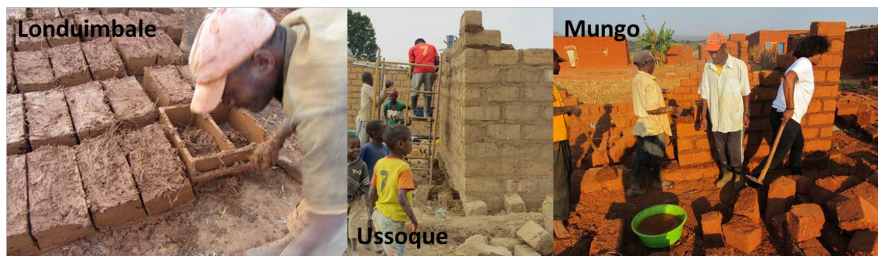
Figure 4 – Manufacture of adobes in Huambo Province - Angola.
