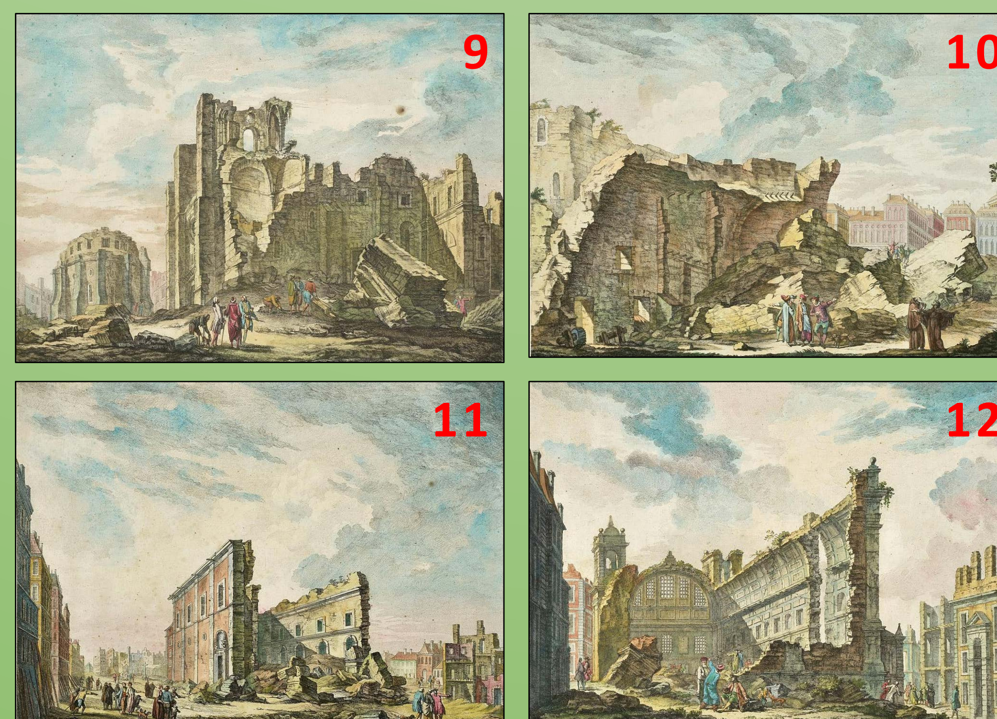
Engravings made by Jacques Philippe Le Bas on 1757 illustrating damage caused by the 1755 Great Lisbon earthquake showing the Lisbon Cathedral (9), the St. Roch Tower (10), St. Paul's Church (11) and the St. Nicholas Church (12). The roofs of the studied buildings partially collapsed along the vertical direction and within their own footprint indicating the prevalence of the vertical component.
