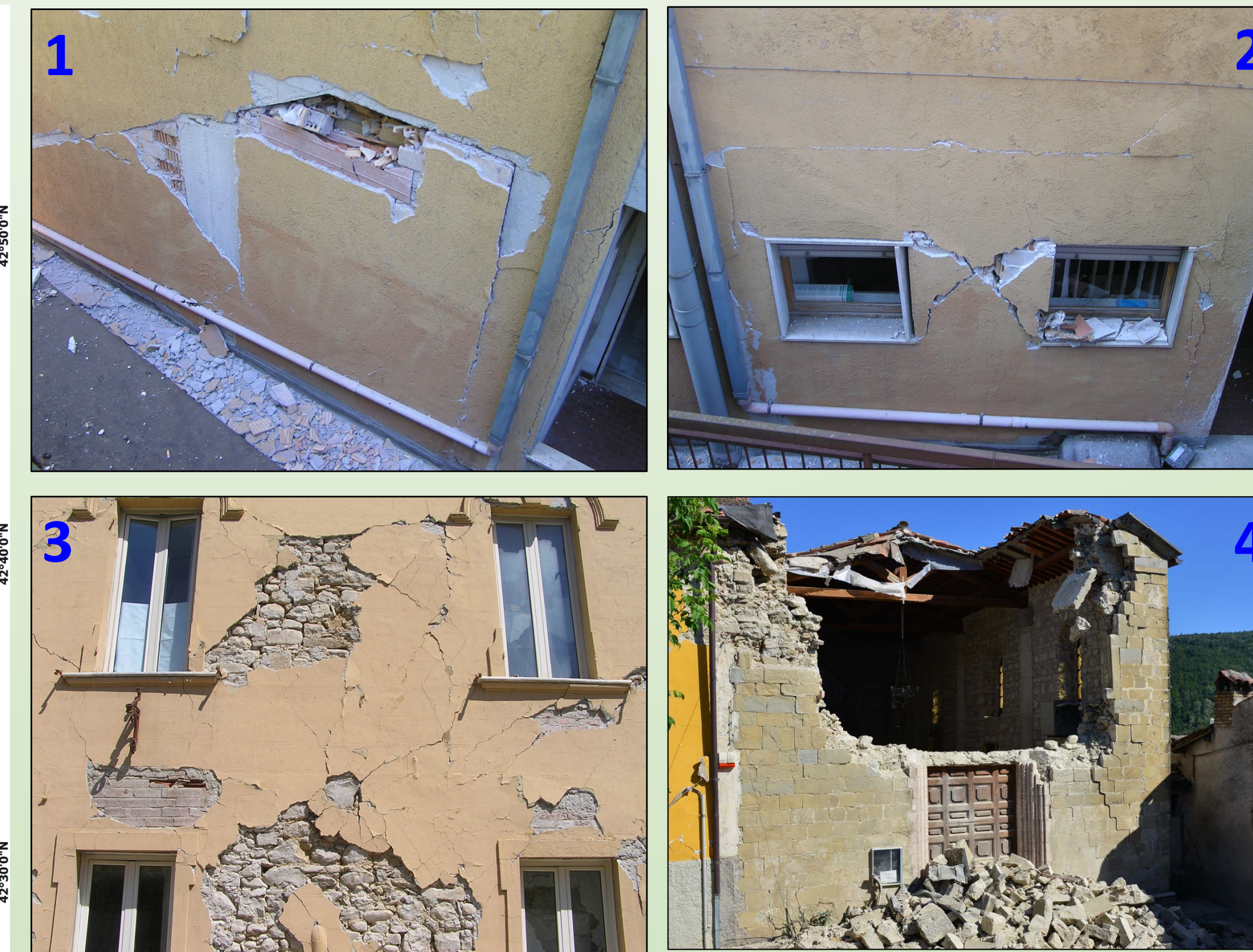
(1, 2) Non-structural damage observed in reinforced-concrete (RC) buildings in Amatrice town. (3, 4) Non-structural and structural damage to unreinforced masonry (URM) buildings in Amatrice (3) and Accumoli (4) towns. Both towns are located close to the causative fault of Mt. Vettore.
