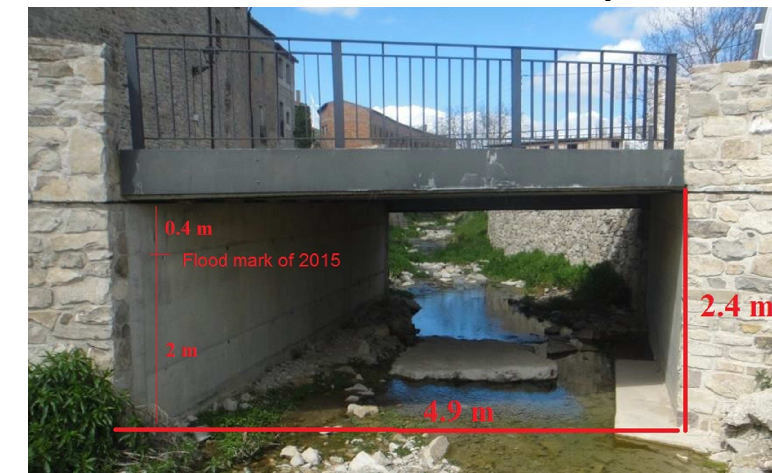
Figure 5. Mark of 2015 flood at Riera de les Hortes and Riera de la Canal junction (see Figure 3)
