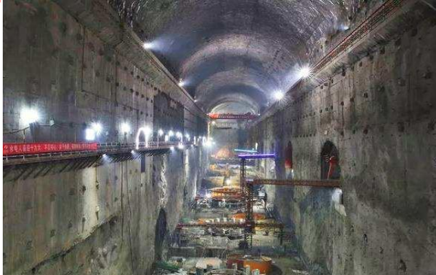
WuDongDe main powerhouse: L \times H \times W = 333 \times 90 \times 30.5\text{m}
