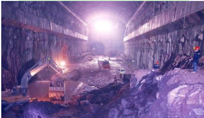
HuangDeng main powerhouse: L \times H \times W = 228 \times 76 \times 33\text{m}
