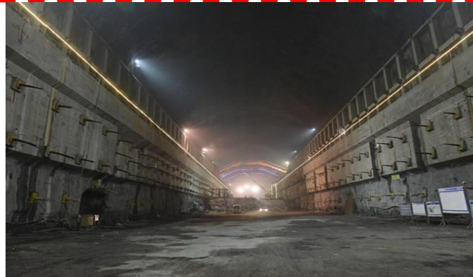
Baihetan main powerhouse: L \times H \times W = 438 \times 88 \times 31\text{m}
