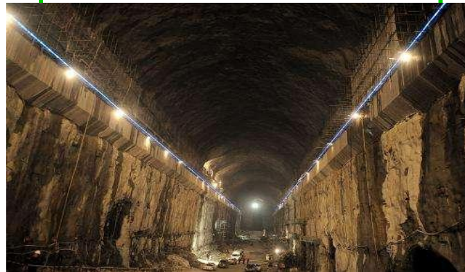
JinPing main powerhouse: L \times H \times W = 276 \times 68 \times 25\text{m}
