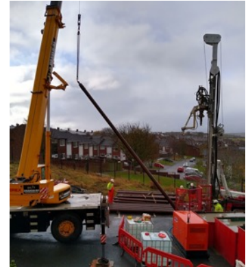
Drilling injection bore hole at Louisa Centre, Nov 2019
