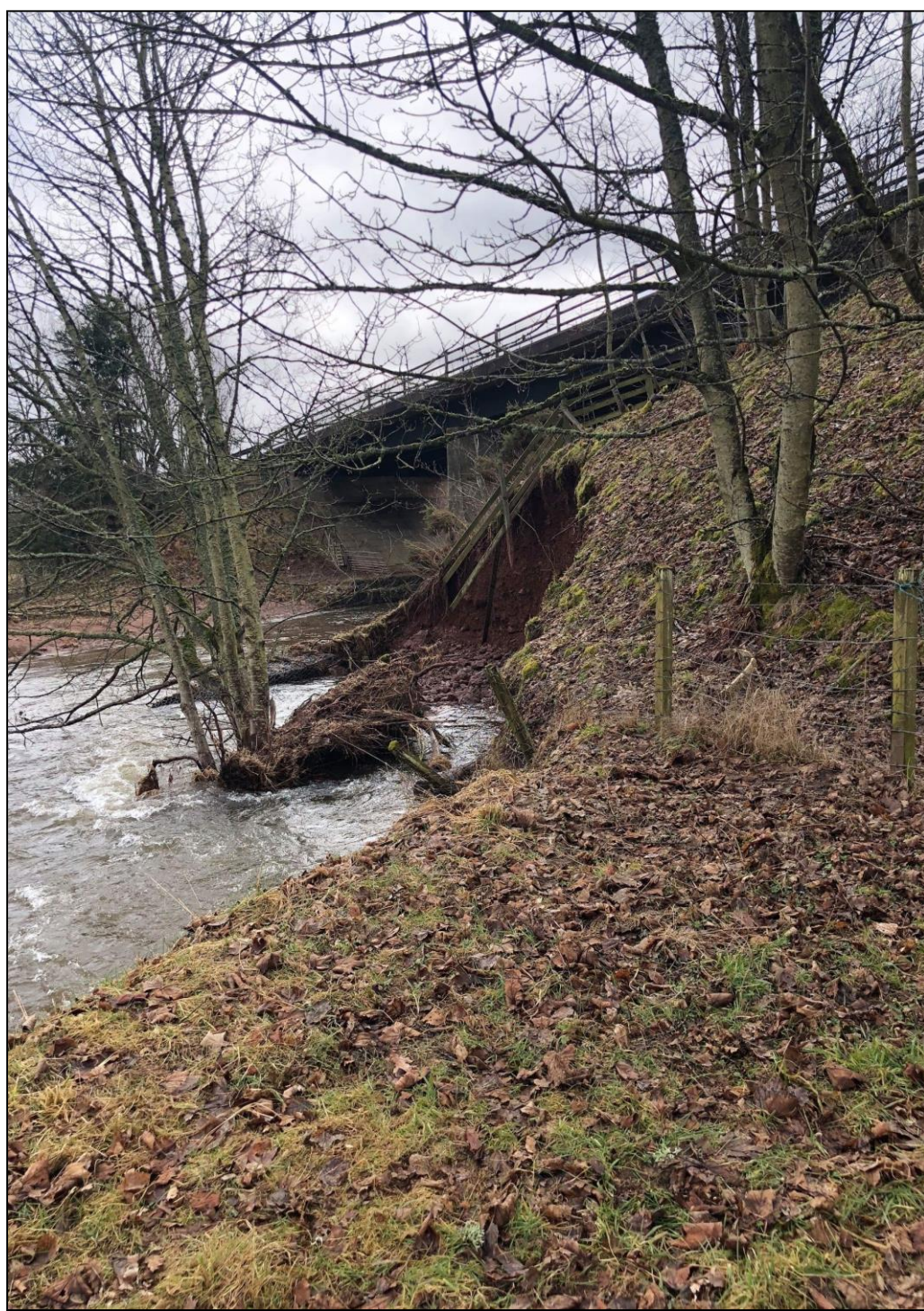
Figure 5 Eroded Embankment (Mar 2018)
