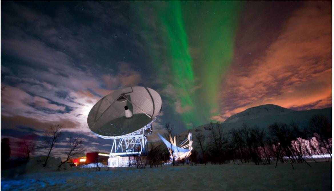
**Figure:** The EISCAT facility outside Trømsø. In the front is the UHF radar used in this study, which operates in the 931 MHz band.
