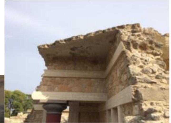
Deterioration of concrete in reinforced concrete elements built during the restoration by Sir Arthur Evans .
