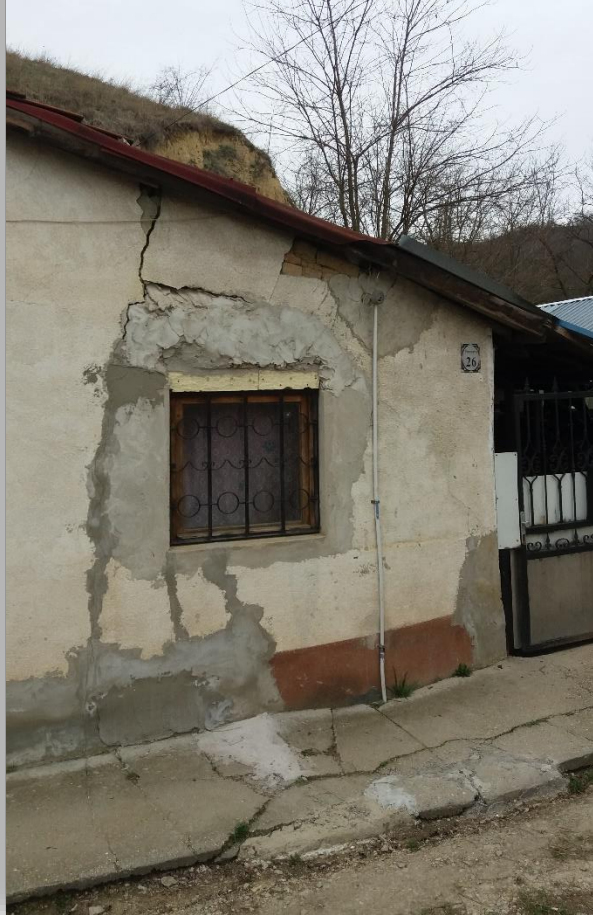
Damaged house built above landslide scarp (Sárisáp)
