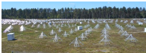
Figure 3: The NenuFAR radiotelescope under deployment, with >1000 antennas already installed.
