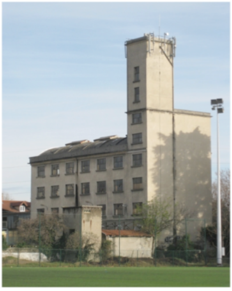
Figure 2: The old factory "Les moulins de Villancourt"
