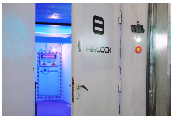
Fig. 2. Airlock module connecting the habitat with EVA terrain. Sterilization area with UV light is activated every time whenever doors are opened. Green and red signaling for “stop” and “go” commands are both located inside the habitat and in the airlock (photos: Space Garden).
