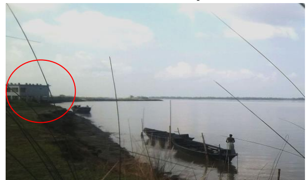
Figure 8. Govt. Primary School at Belgacha facing serious threat of bank erosion .
