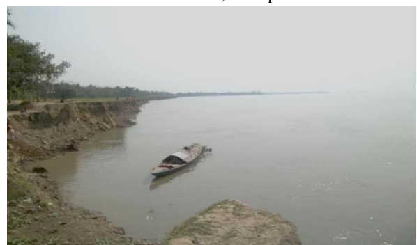
Figure 10. Bank erosion 6 km south from Bahadurabad.
