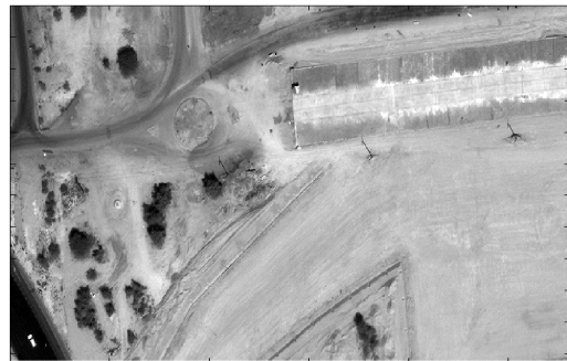
Figure 4. Right Pleiades satellite stereo image contains four power poles and vegetation near power two poles
